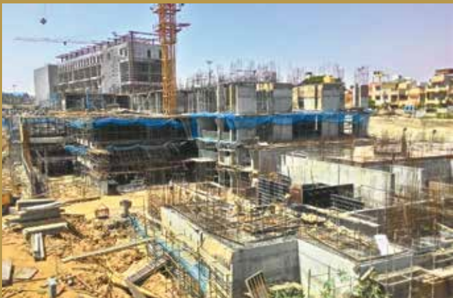
Glen Classic Excavation
